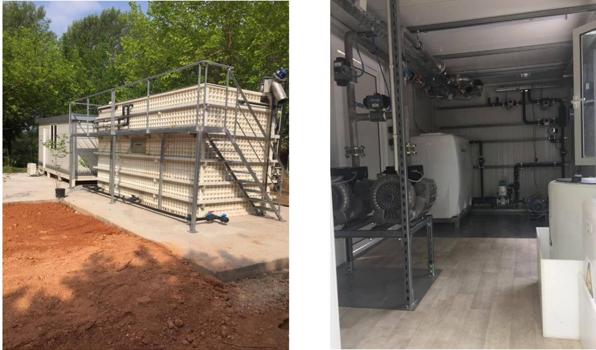
**Figure 3.** Images of the MBR used in NextGen project.
