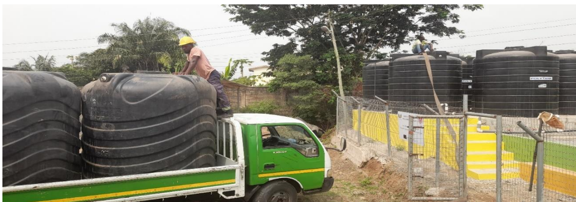
Figure 6: Discharge of water from SSGL RAW water into polytank
