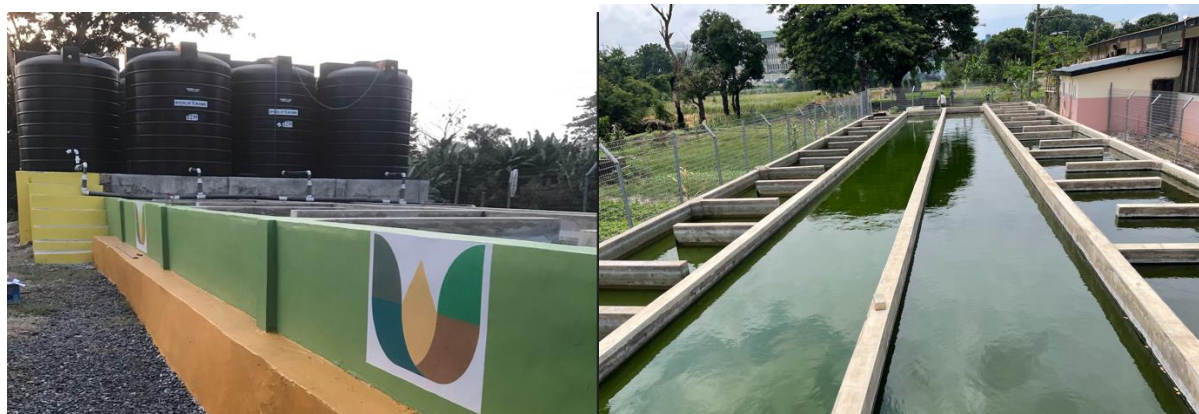
Figure 7: Reservoir with baffles
