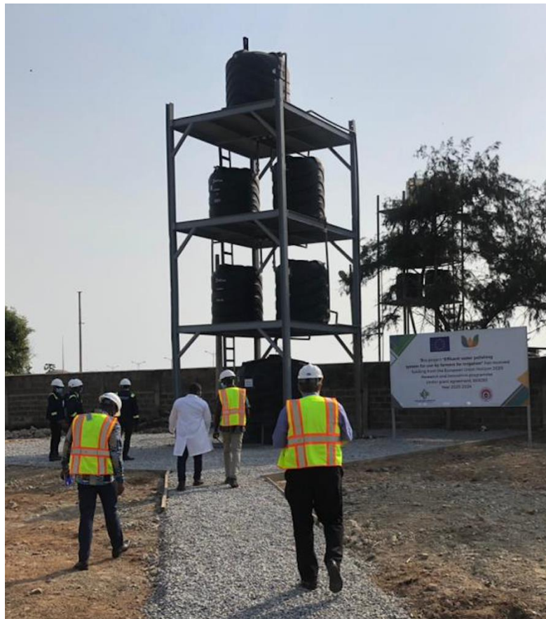
Figure 2: Filtration system at SSSL
